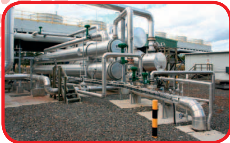
Eastland Group's 9 megawatt power station KA24 at Kawerau.
